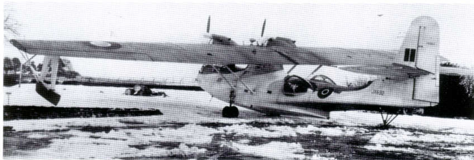
► PB2B-2 — one of several used by the US Navy. This had the Nomad tail, radar radome, and “Eyeball” turret plus de-icing system / National Archives
