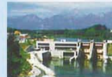
Elektrownia wodna Mavcice Mavcice hydroelectric power plant 200 MW
