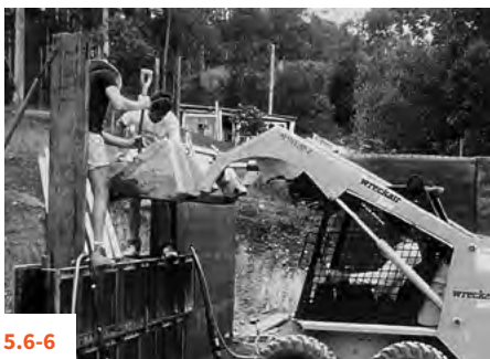
5.6-6 | 5.6-7 MECHANICZNA GLINOBITKA, TERRASTONE, AUSTRALIA
